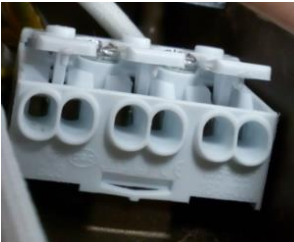
Figure 4. Terminal block
